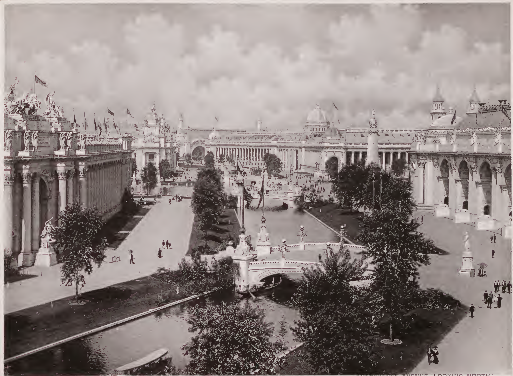
TRANSVERSE AVENUE, LOOKING NORTH.
